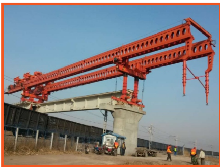
Launching Girder (Metro)
