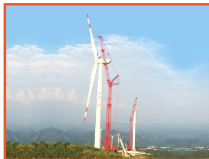
Wind Mill Crane
