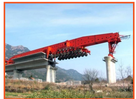
Launching Girder (Bullet Train)
