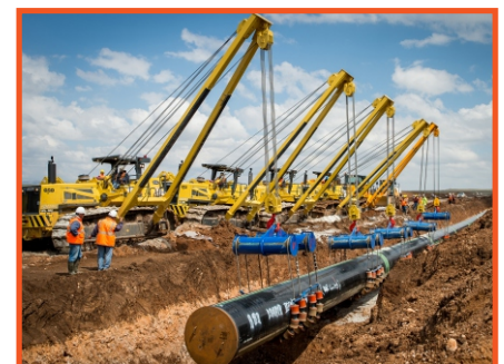
Pipe Layer & Pay Welder
